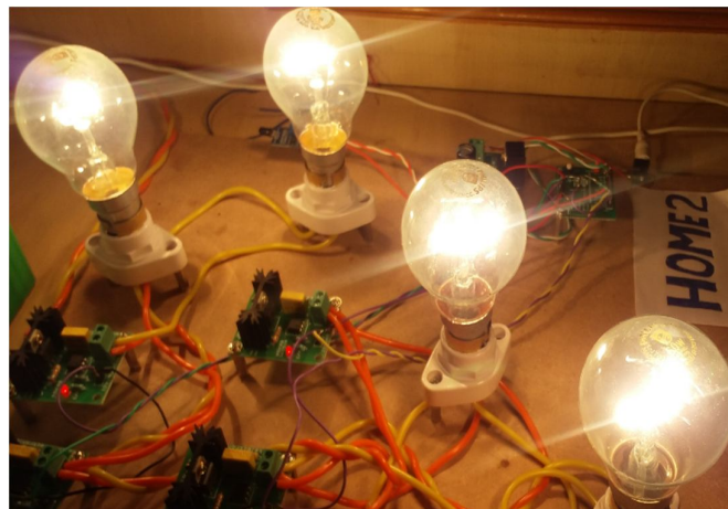
Fig.3. Test bed with four loads connected to it
